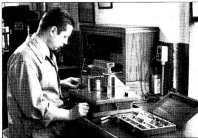
Fig. 2. Below—Checking a Fixture with Precision Gauge Blocks
