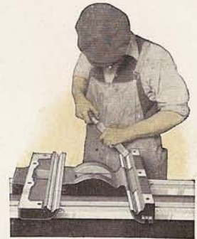
Fig. 19. Hand Scraping Cross Slide to Bed
