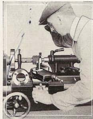
Cutting a Screw Thread
