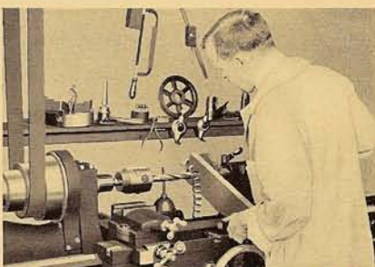
Fig. 8. Lathe Used as Drill Press for Drilling Hole in Flat Piece of Work.
