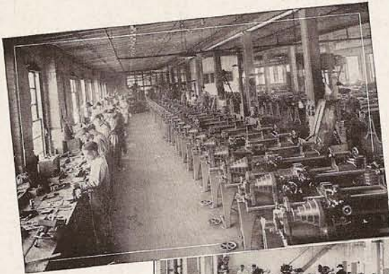
Above—A view of the Assembling Line where 25 Lathes of one size are assembled at one time.
