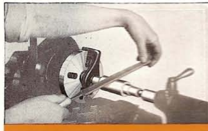
Fig. 39. Lathe is Practical for Filing and Polishing Bushings, Shafts, Parts, etc.
