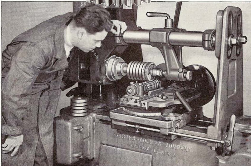
Fig. 27. One of 21 Automatic Gear Hobbing Machines in the Gear Cutting Department.
