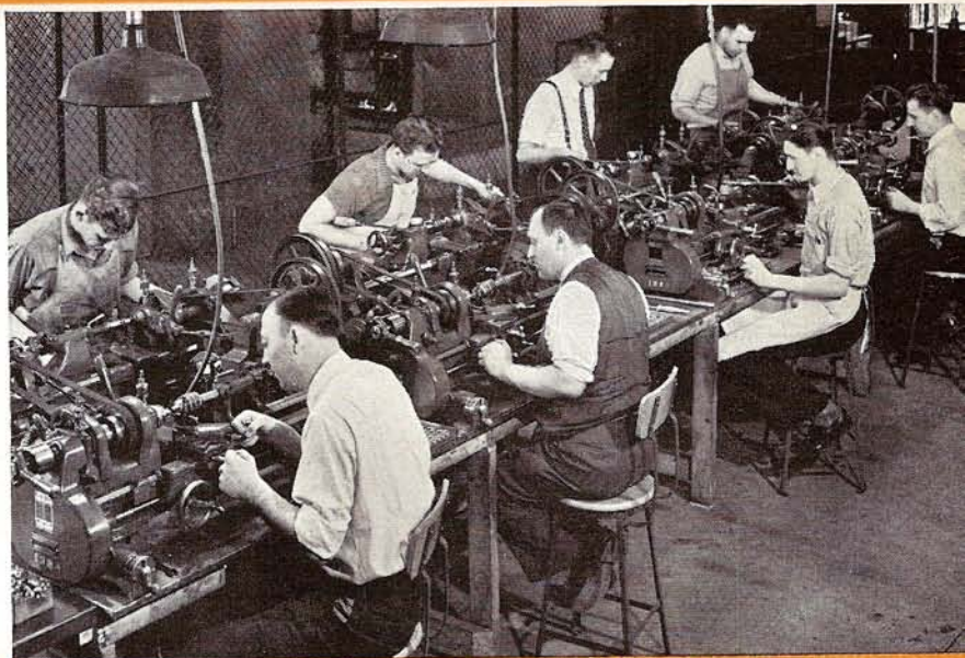
Fig. 90. A Battery of Eight "Workshop" Bench Lathes in a Radio Factory.
