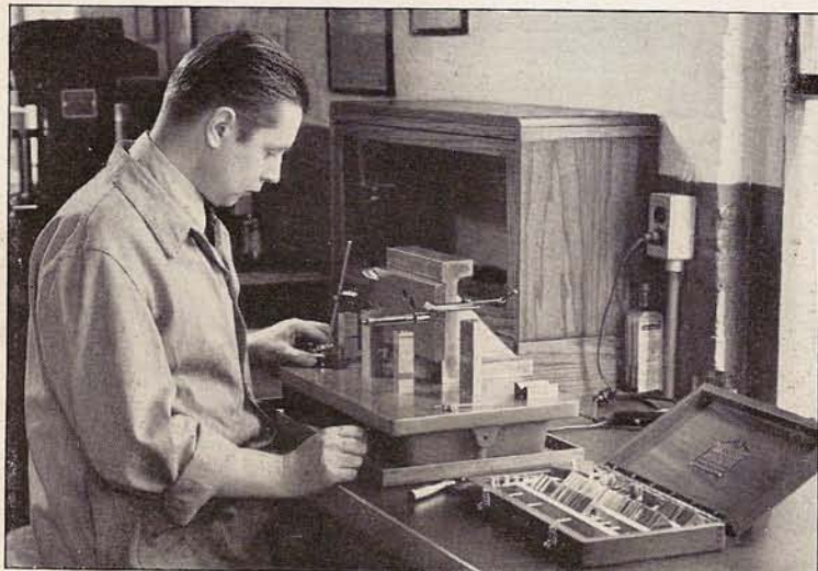
Fig. 2. Below—Checking a Fixture with Precision Gauge Blocks
