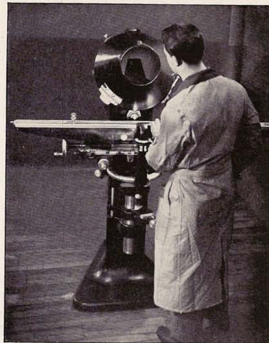
Fig. 3. Inspecting a Screw Thread with an Optical Comparator
