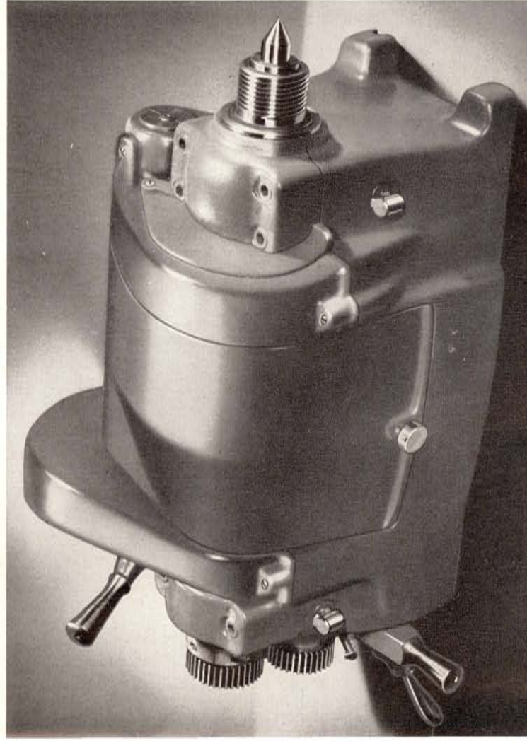
Fig. 13. Left—Headstock for 16" South Bend Lathe
