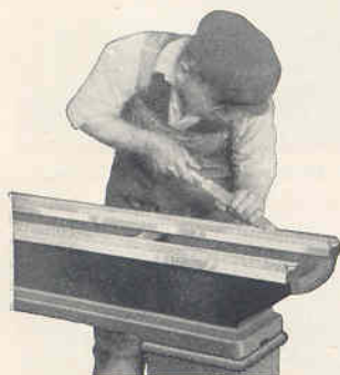
Fig. 35. Hand scraping the V-ways and Flat-way of the lathe bed.
