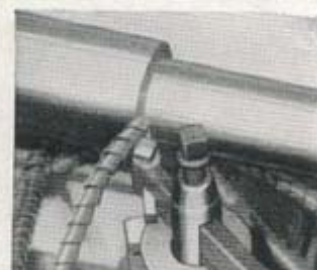
Reducing a cold rolled steel shaft from 3 1/2 to 3 inches.
