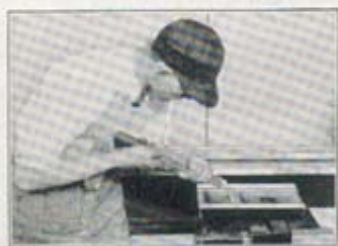
Hand scraping base of Tailstock.
