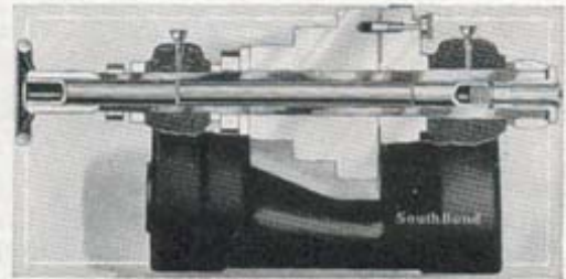
Cross Section of Headstock showing Draw-in Collet Chuck
