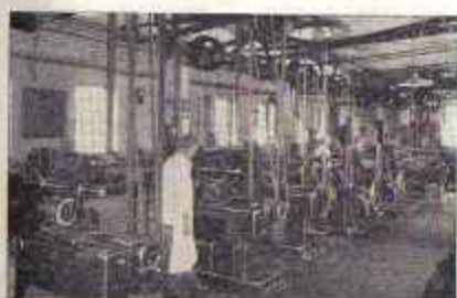
Fig. 91. Gear Cutting Department
