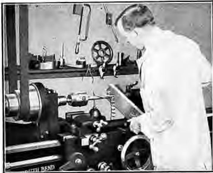
Fig. 619.—Operation of a Drilling Job
