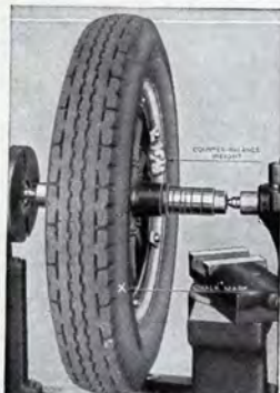
Fig. 630.—Balancing an Automobile Wheel
