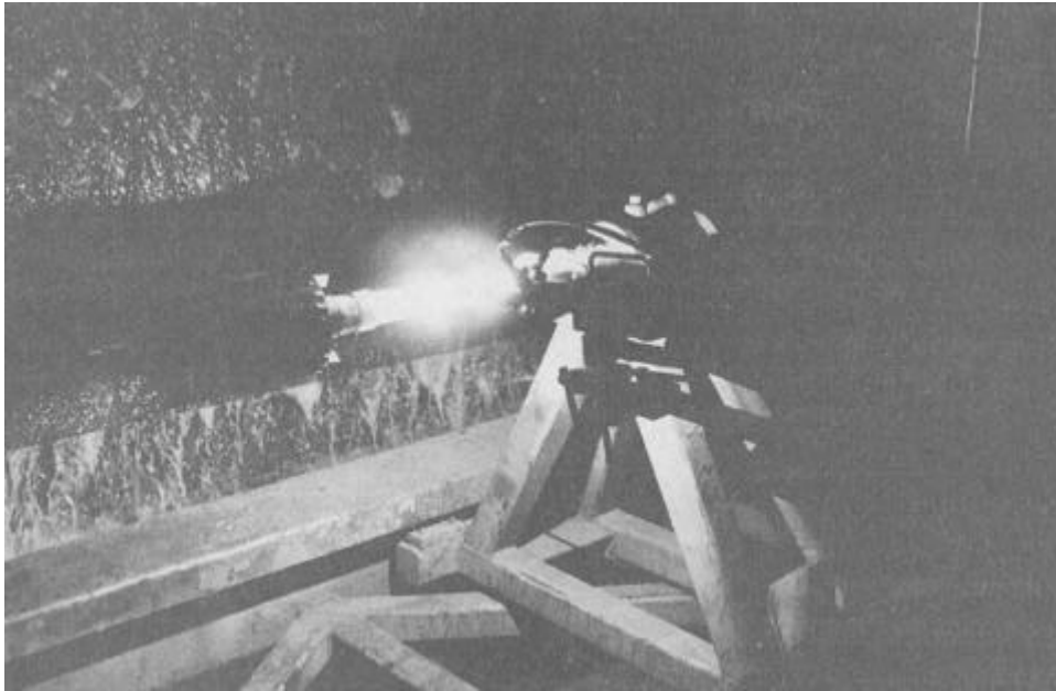
Figure 12-9.—A shaft being thermal sprayed.
