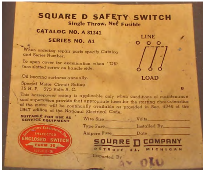
Figure 98: Notice page inside safety switch.
